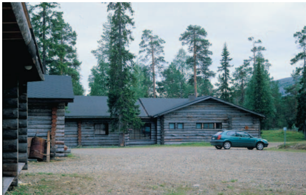
Fig. 2. Kelo offers excellent timber for building; its grey colour comes from blue-stain fungi. The oldest part of the Luosto Reserve headquarters was built in 1971 when kelo was common in the area in many kinds of forests. Finland, Sompion Lappi prov., Sodankylä, August 1998.
